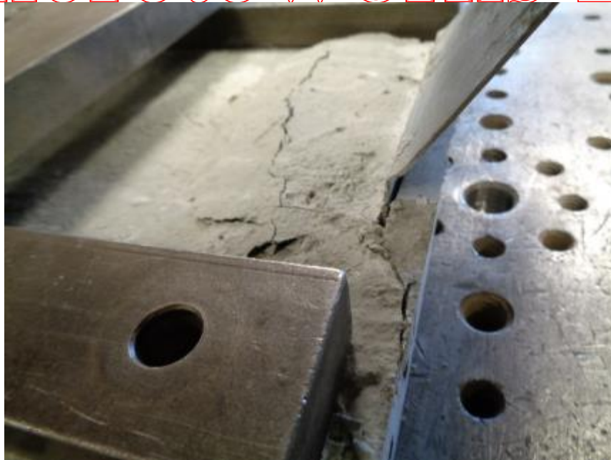
Photo No. 8 ASTM E488 Shear - Embedded Mechanical Clips Failure Mode
